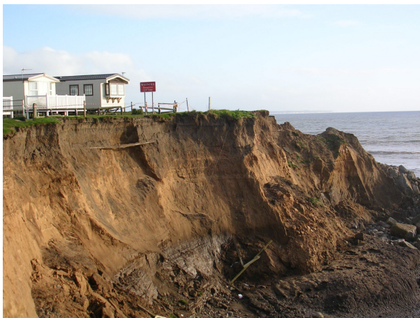
Figure 9: Cliff collapse at Barmston, Yorkshire (Peter Kennett)
